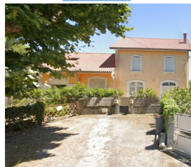
Figure 33 : Ancienne gare. Source : google street view
